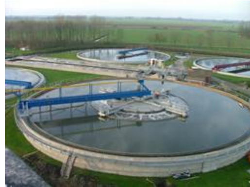
Figure 1: The clarifier at the wastewater treatment plant.
