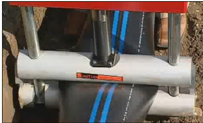
Figure 1. Squeeze-off of PE pipe
