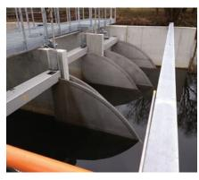
**FIGURE 3.** View of the adjustable dam at the outlet of the aeration channel.
