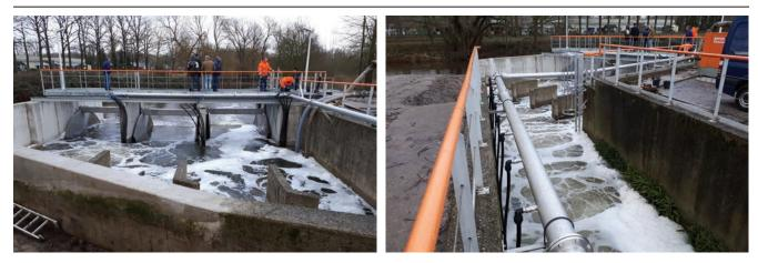
FIGURE 7. The aeration channel of the Eindhoven Wastewater Treatment Plant in full operation as it improves the oxygen quality of the effluent before reentering the Dommel. Left: View of the adjustable dam at the outlet of the aeration channel. Right: View of the aeration channel from the inlet.
